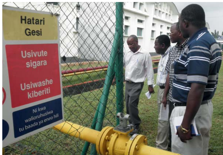
Natural gas infrastructure at Tanzania Cigarette Company Limited in Dar es Salaam. A Cost of Service Study (COSS) to establish costs involved in generation of electricity from gas after completion of a bigger gas pipeline will be instituted.
