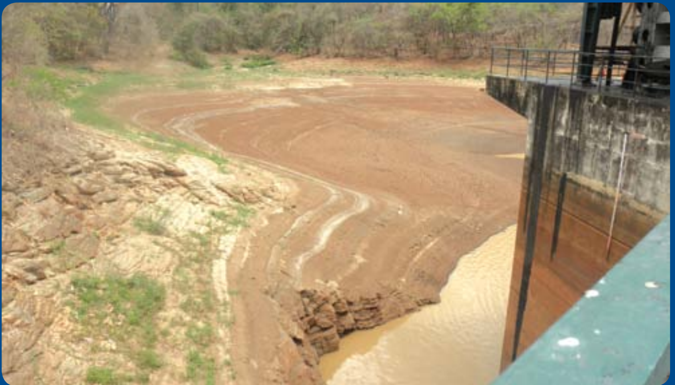
A section of Kidatu Hydro Dam in a photo that was taken on 14th September 2012 , showing diminished water levels that have affected power generation in the country.
