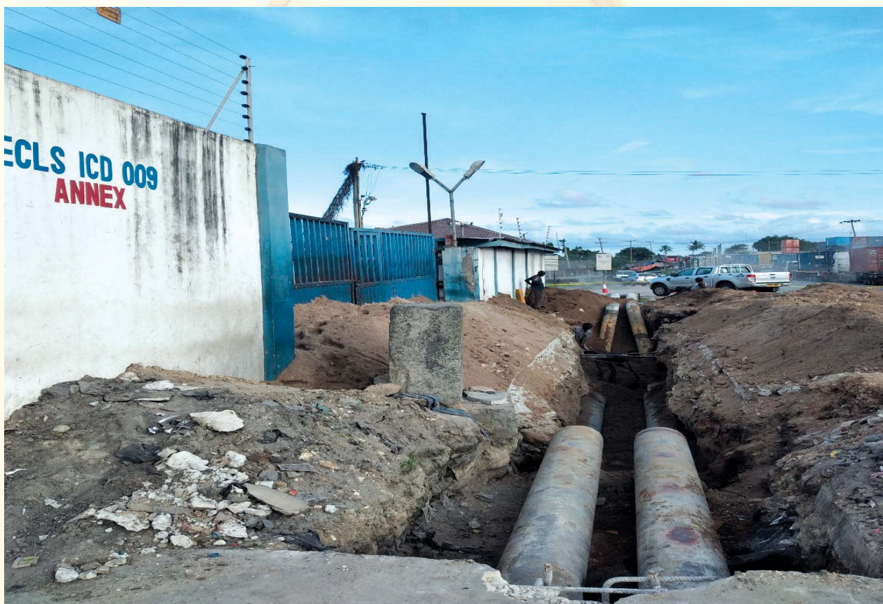
Figure 33: Exposed underground pipelines crossing ICD entrance gate at Kitopeni area in Dar es Salaam.
