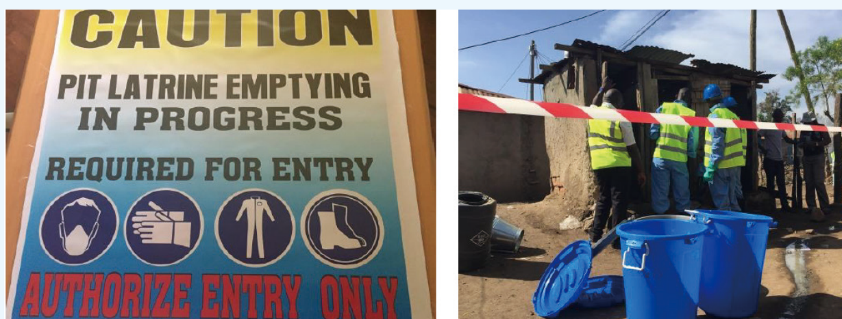
Figure 4- 6: Sample hazardous workspace signage (Left), Barrier tape erected around workspace (right).
